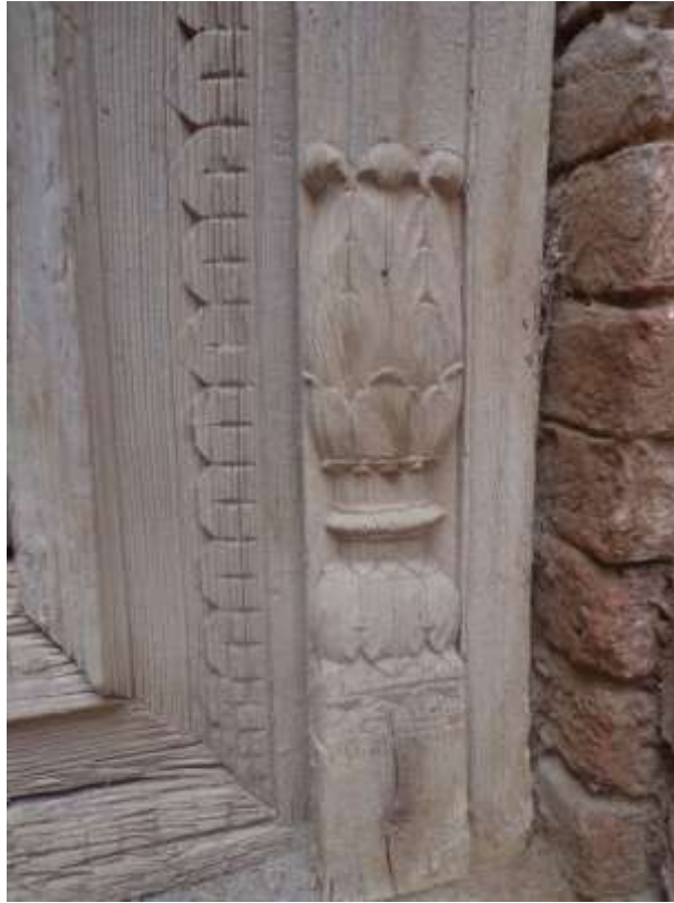
Plate.9. Carved patterns on both sides of wooden frame of door. Image by Researcher.
